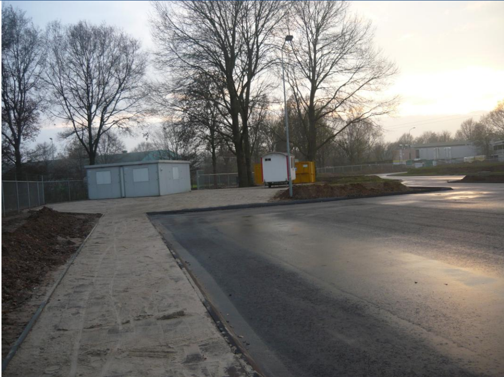
De verharding is gereed...
